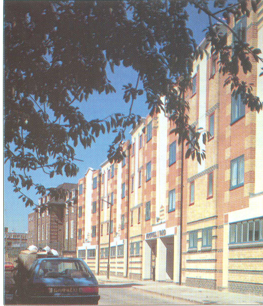
Front elevation and main entrance.
